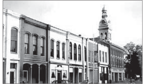
Nicholasville, Wilmore and Jessamine County firefighters worked together in an attempt to save this historic block in December 2004.
